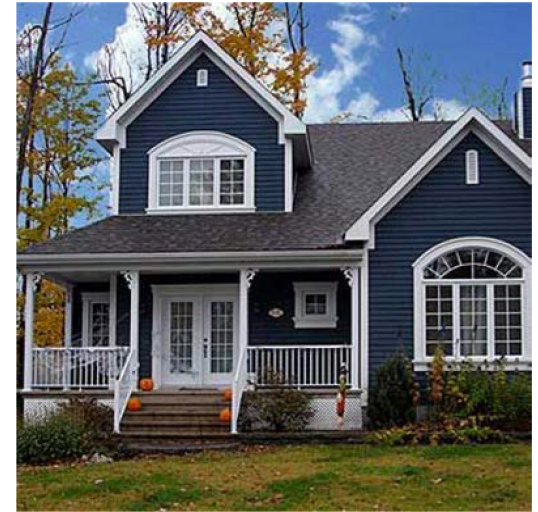
Door, Windows, Steps
